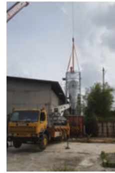
The furnace for the new cyclone system.
